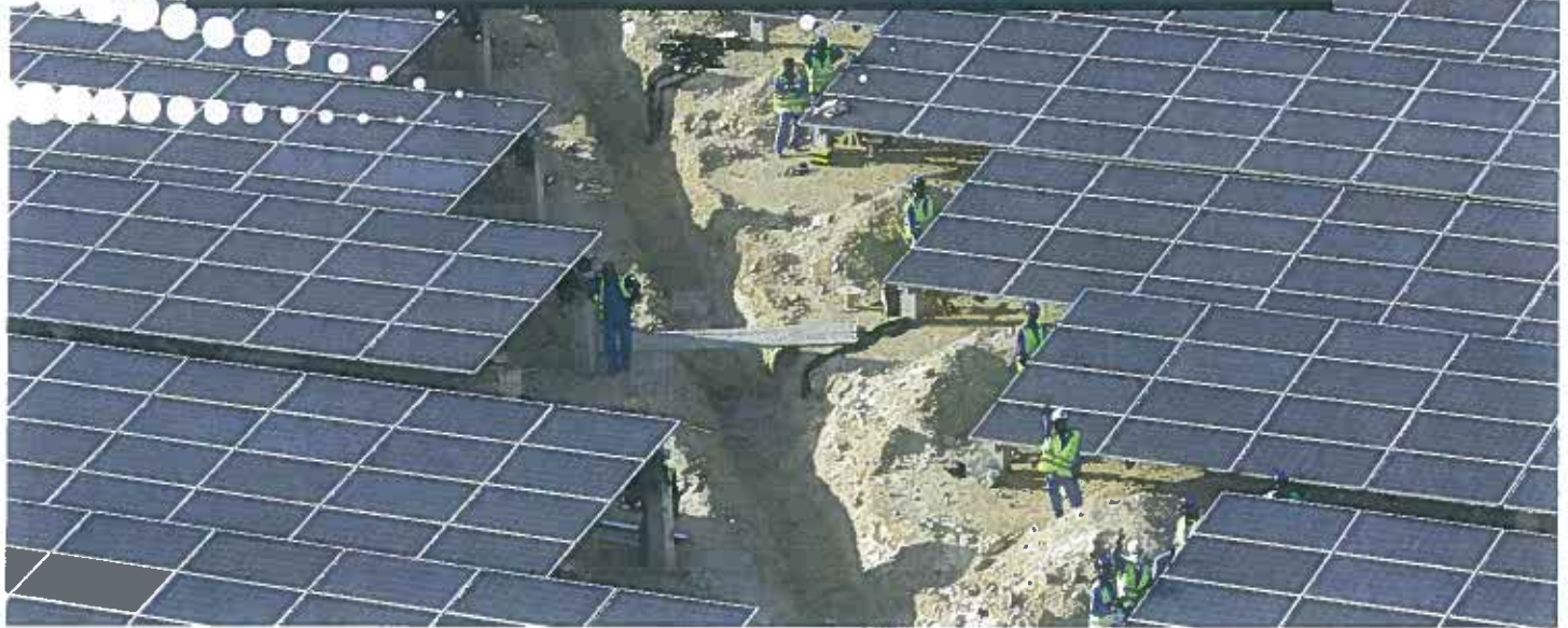
▲ Thin Film modules (left) line up next to the smaller crystalline modules (right).
